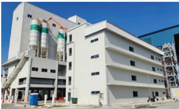
Island Concrete commenced operations at its at Jurong Port's Ready-Mixed Concrete (RMC) Port-Centric Ecosystem. It is Singapore's largest concrete batching facility at the multi-purpose port that improves environmental sustainability and operational productivity by integrating raw materials like cement and aggregates to reduce number of truck trips required.
