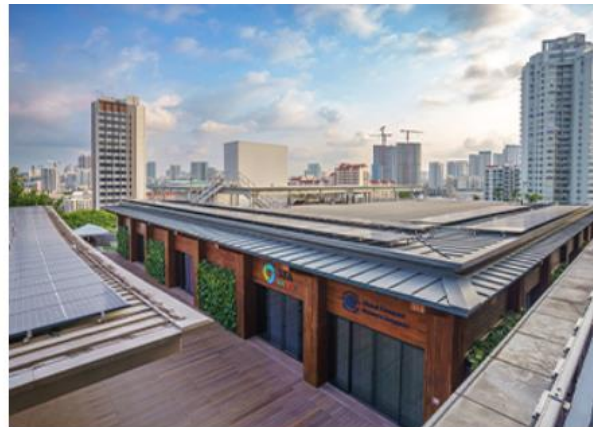
Designed for climate resilience, the SSA Annex is powered by a 31.6 kilowatt peak (kWp) rooftop Solar Photovoltaic (PV) System enabling it to achieve net-zero operational energy.
