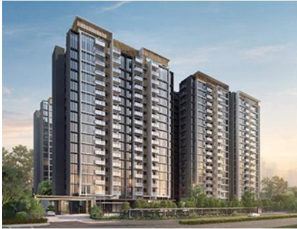
The 566-unit Penrose is a joint development with CDL located in Singapore's east side at Sims Drive. It was launched in 2020 and expected to complete next year, 2025. (artist's impression)
