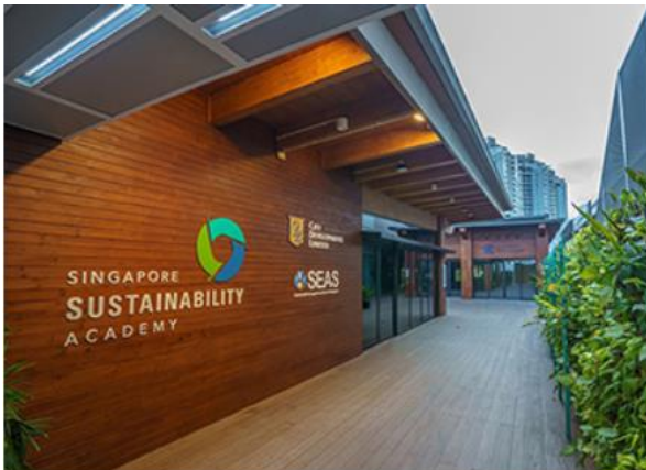
The SSA opened seven years ago on the roof terrace of City Square Mall as a first-of-its-kind hub for sustainability education and action.
