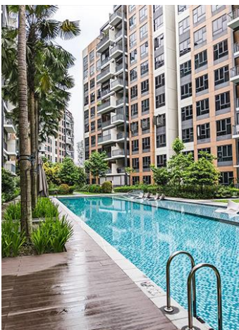
CDL was the first developer in Asia to adopt Prefabricated Prefinished Volumetric Construction (PPVC) for a large-scale residential development. (Pictured: Brownstone Executive Condominium launched in 2015).
