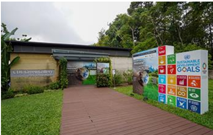
The 3,3809 sq ft CDL Green Gallery is an eco-friendly building built with bio-composite material Hempcrete, and a prefabricated modular system that reduced on-site construction time to under 24 hours. In July 2021, CDL opened the first instalment of its three-part climate action exhibition series, "Change the Present, Save the Future" to support both global and national climate efforts.
